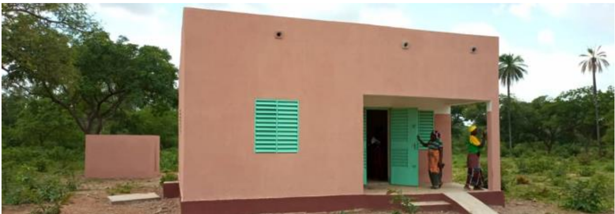
A staff house at the medical center Sipigui
