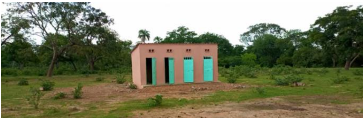
Latrines at the medical center Sipigui
